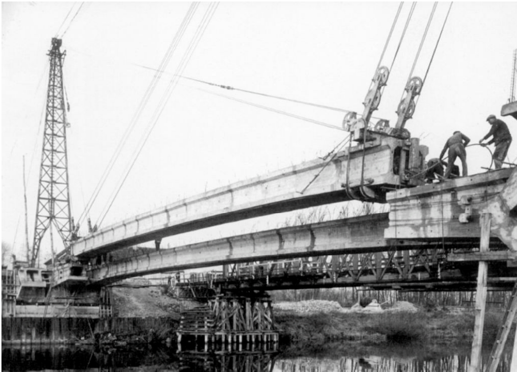
Figure 16 - Luzancy Bridge segment erection
