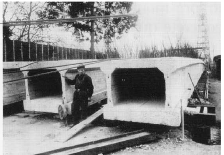
Figure 15 - Luzancy Bridge segment assembly
