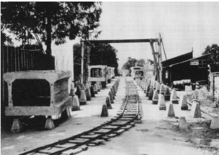
Figure 14 - Luzancy Bridge segment casting
