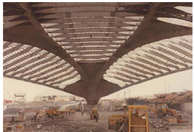
decentered structure (564 ft span)
