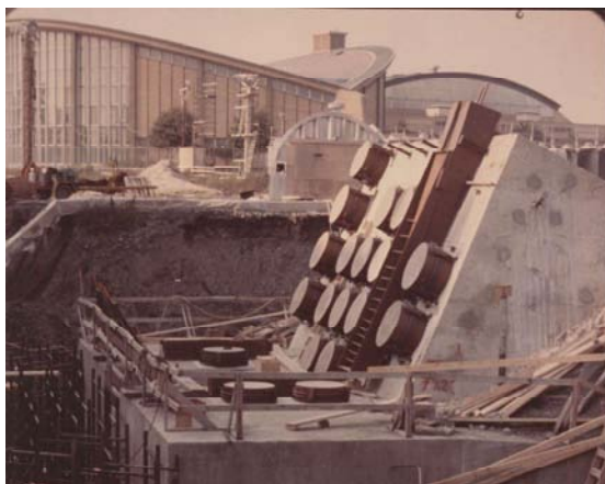
flat jack layout at abutment Z
