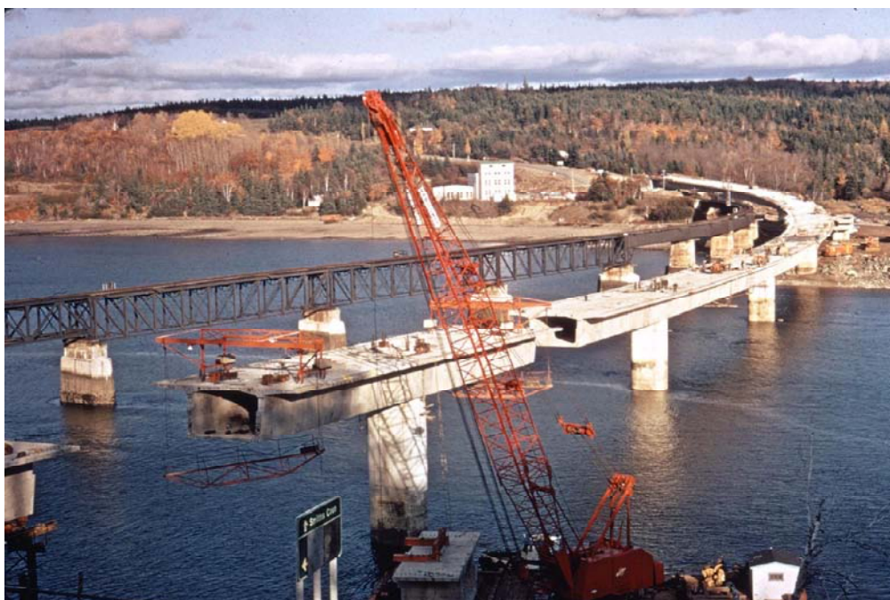
Figure 19 - Bear River Bridge (1971-1972) (first precast segmental "match-cast" bridge in North America)
