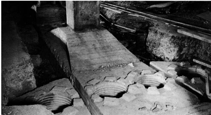
Figure 12 - Le Havre existing columns above and new piles below footing
